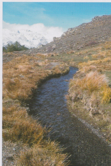
Ancient Acequia: hand dug irrigation ditch carrying water from the Sierra Nevada to the fields below.
